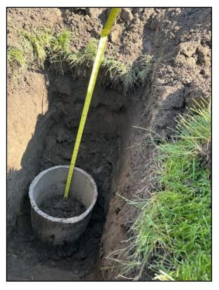
PHOTO 17: HOLE 3 FEET DEEP, 12X24 RING, 10 INCH ABOVE GROUND. 14" OF EMBEDMENT.
