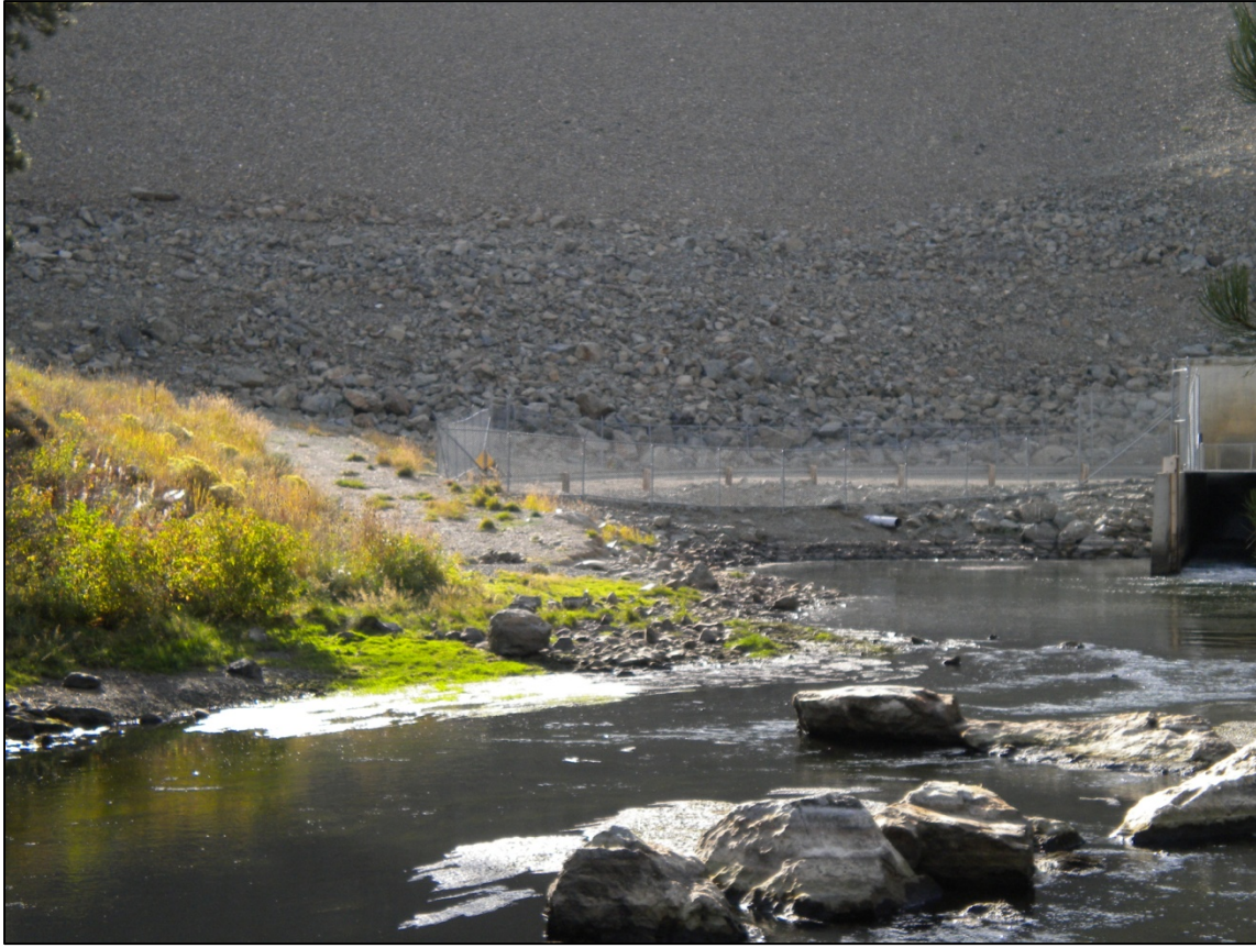
FIGURE 16. PHOTOGRAPH OF SOUTH BANK OF MASON DAM TAILRACE POOL SHOWING LIMIT OF POWDER RIVER RIPARIAN ZONE.
