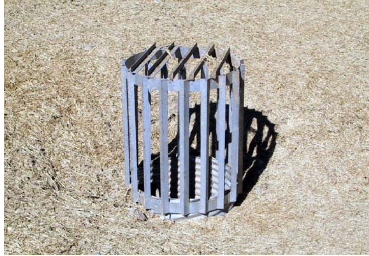
Figure 1. Metal trash rack used to protect drop inlet
