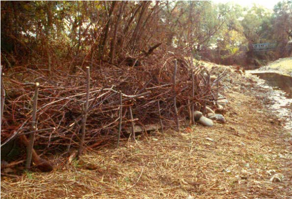
This brush box was made using mostly dead plant materials, and was intended to protect this eroding streambank and encourage siltation.
