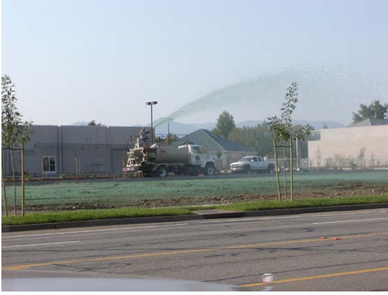
Hydroseeding site in September 2003
