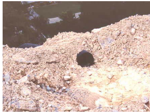
Figure 2. Diversion dike used in combination with a flexible slope drain
